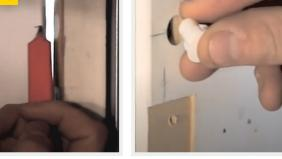
Align the DPS location onto the door jamb using a pencil. Drill a 12.5mm diameter x 15mm deep hole. Fit the DPS magnet into the door jamb. Mark the position of the latch bolt to determine the striker height. Fix the strike box to the jamb and then secure the strike plate over with the timber fixing screws. For lock setup, please refer to the Yale Home Quickstart Guide.
