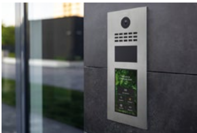
Main entrance: D31TDV IP video door intercom system including RFID, Bluetooth, keypad, and QR code scan
